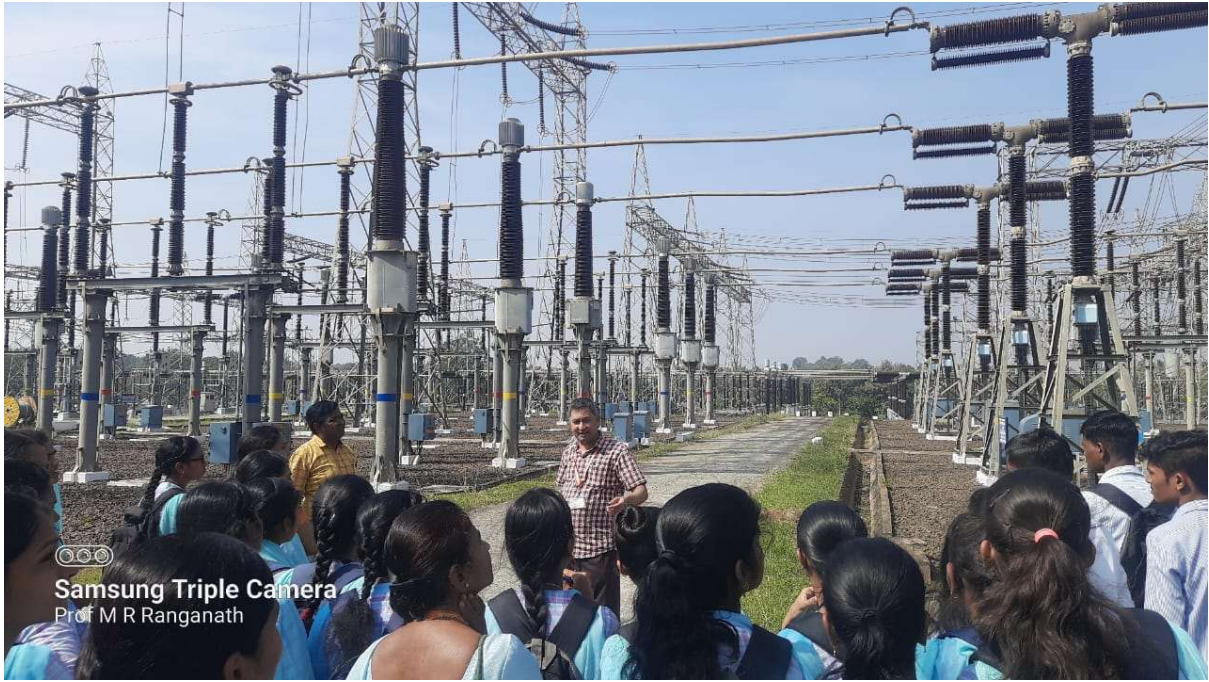
Near the Current Transformer
