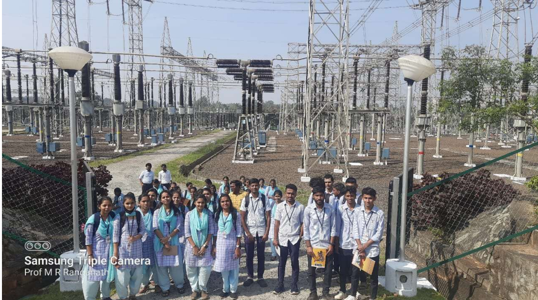
At the Electrical Switchyard
