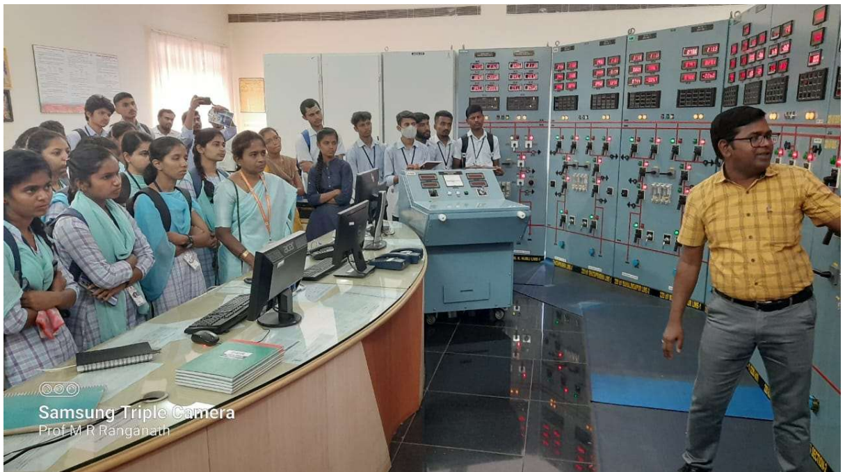
Inside the Control Room
